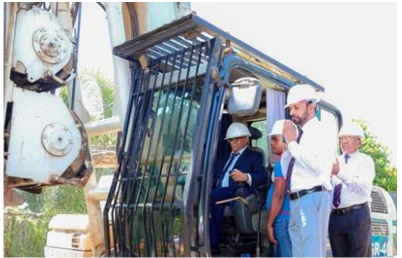
Hon. Minister Anura Karunathilaka starts operating the Piling Rig
