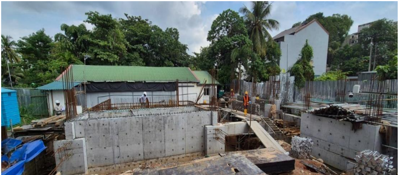
Substructure Structural Works in Progress
