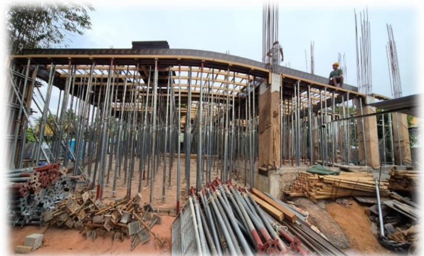
Head Office project – Structural works progressing up to first Floor Slab
