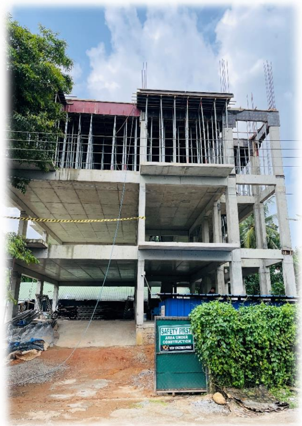
The future Head Office Building of the IIESL in progress
