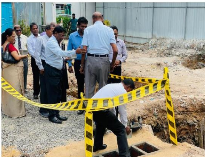
Commencing IIESL Building Construction
