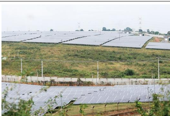
Gannoruwa Solar Power Project in Sri Lanka (150MW) (The Island Online newspaper)
