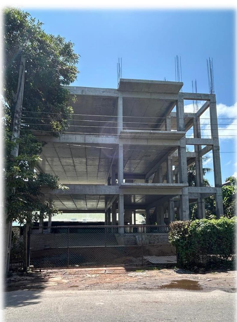
Partly completed, proposed IIESL HO Building
